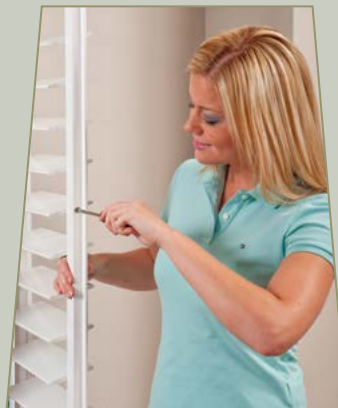
ADJUSTING LOUVER TENSION
