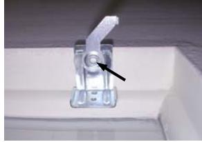
3. Place the headrail against the bracket with the swivel in open position. Then rotate the swivel to a close position. (Check that the headrail is being secured by the bracket).
